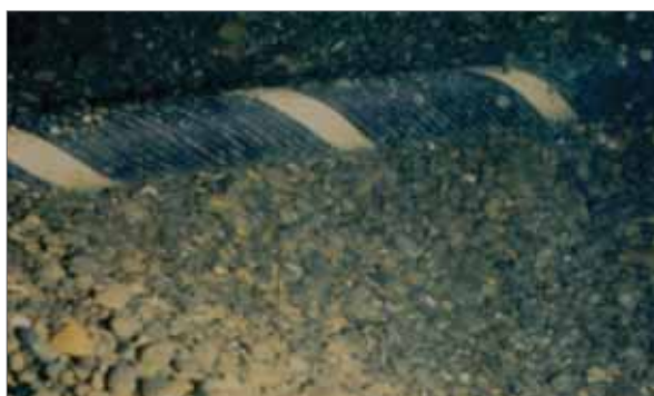
Figure 3.6: Image of a surface-laid cable taken during a post-lay inspection by an ROV. This image reveals the cable in the throes of burial by mobile gravel. Source: Transpower New Zealand and Seaworks.
